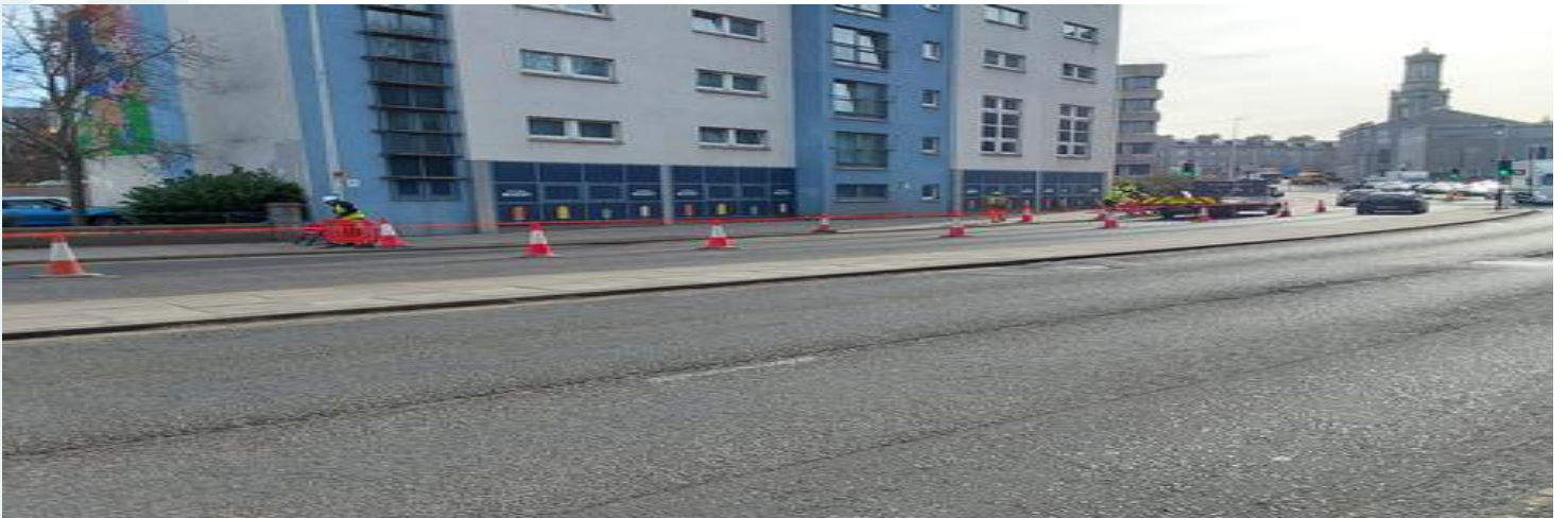
Phase 4 scaffolding lane closure and footpath restrictions.
